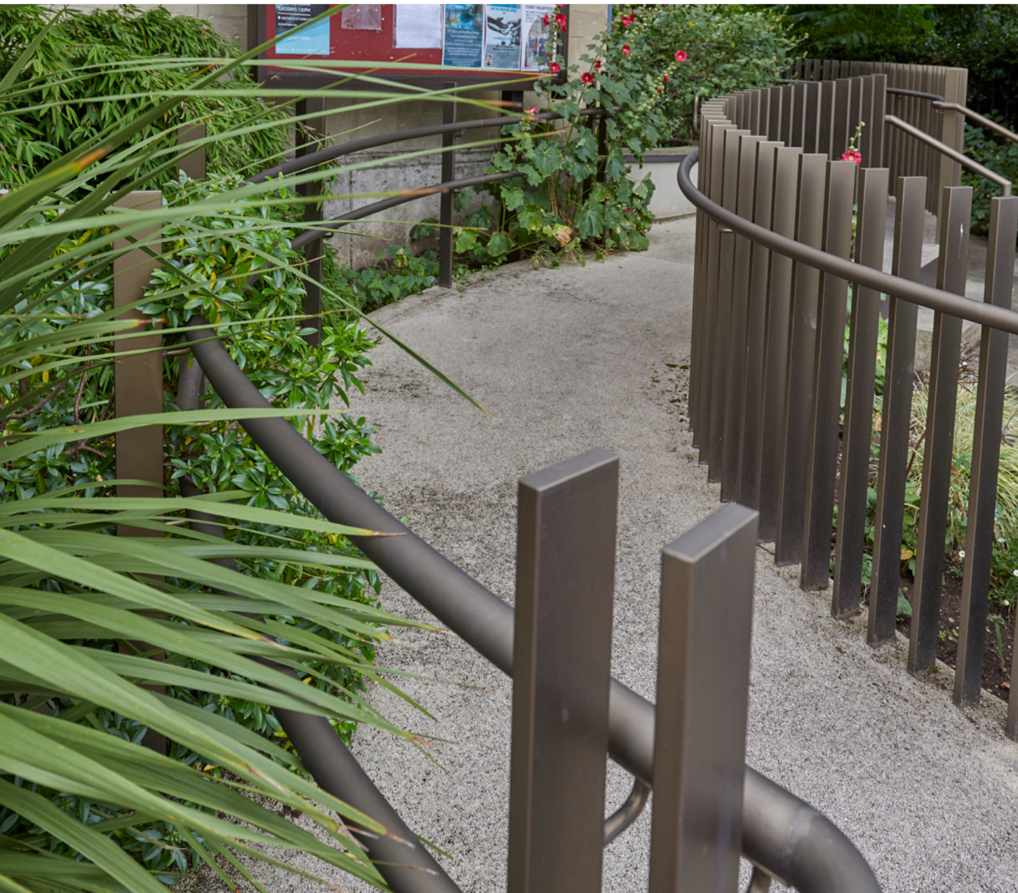
St Mark's Church, Clerkenwell: Ramp installed with funding from Cloudesley
